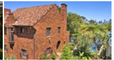
Q4. 88 Wolseley Road, Point Piper $16million*
