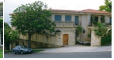
Q2. 63 Wolseley Road, Point Piper $21.5million
