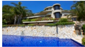
Q1. 110 Wolseley Road, Point Piper $20.6million
