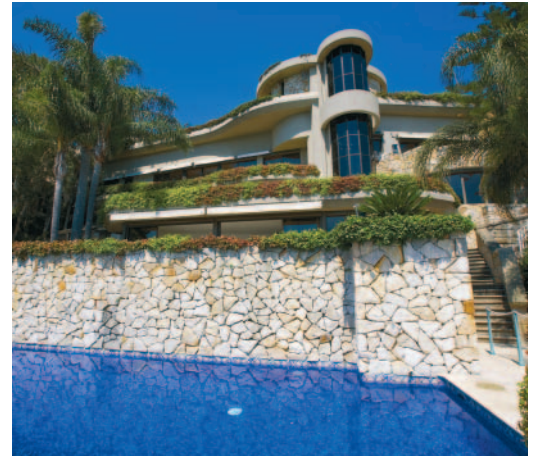
Q1. 110 Wolseley Road, Point Piper $20-21million
